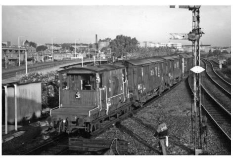
Above: Once over the junction, the train was cleared to reverse from the Down Dalston Main Line by Shunt Ground Signal No 24, which controlled entrance to the run round loop.
