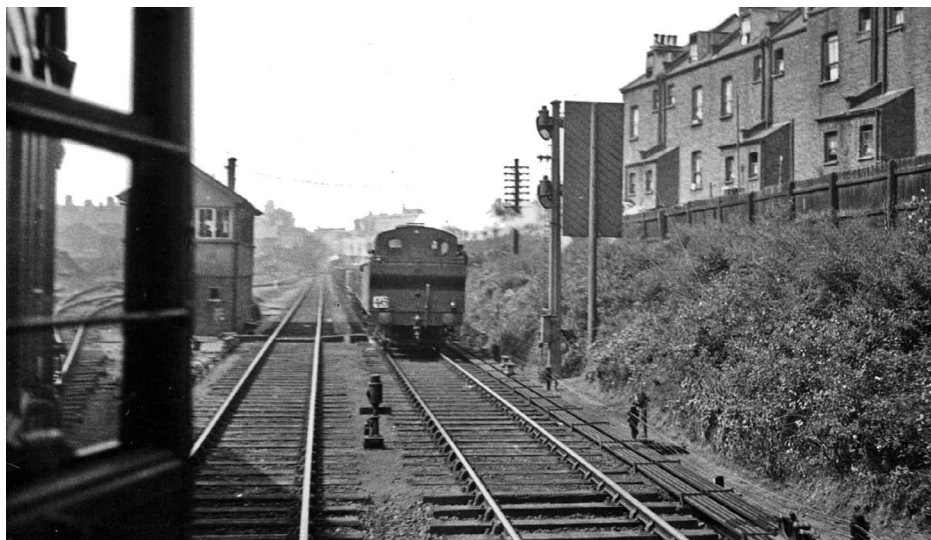
A goods train, hauled by an LMSR Class 3F 0-6-0T, passes the signal box at Dalston Eastern Junction, sometime in the 1920s, with part of Kingsland Yard just visible beyond the open door on the left. Locomotive & General Railway Photographs
